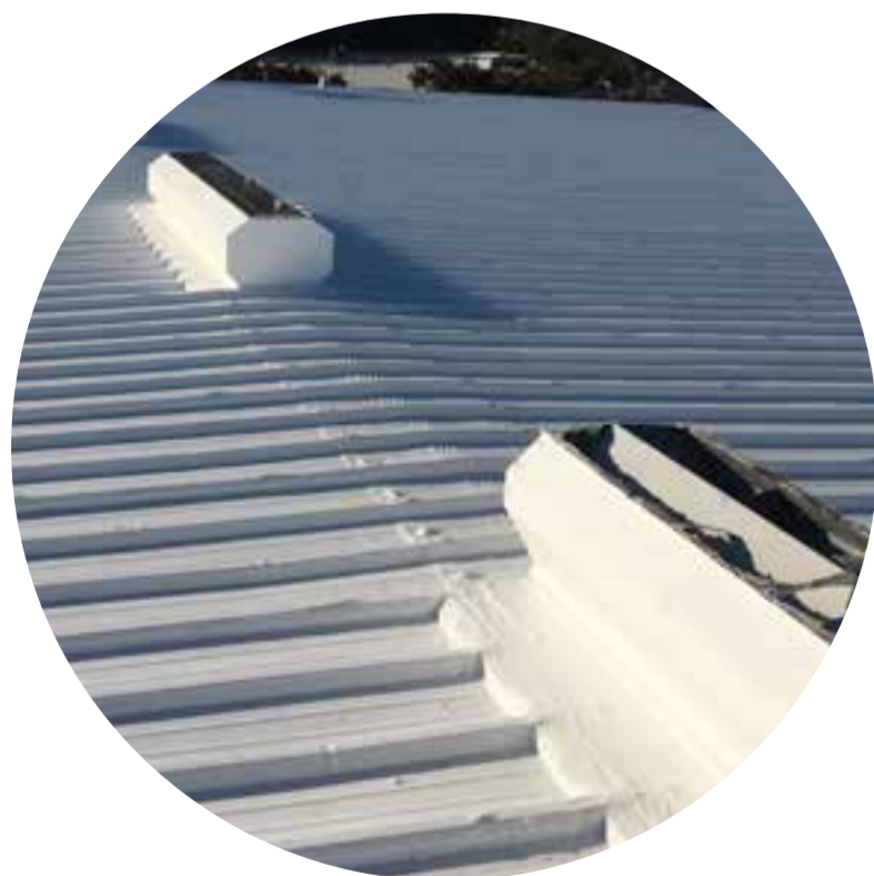
3. METAL OR LOW-SLOPE ROOFING OVER 1-IN-12 VFI-600 Series Acrylic Roofing System
