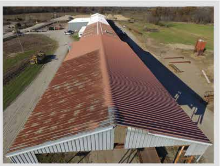
Aerial view of the three step process; Prime, Repair and Coat.
