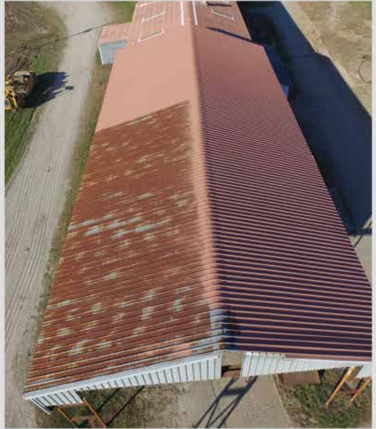
Before and after picture of primed roof featuring VFI-#11 Epoxy Primer
